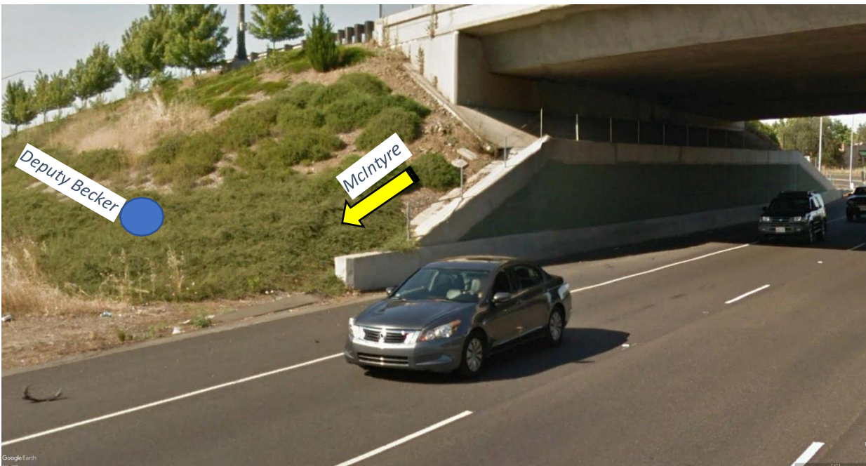
Figure 5- Zinfandel Drive overpass west side
