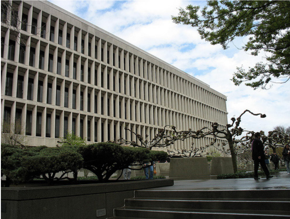
Sacramento County Courthouse
