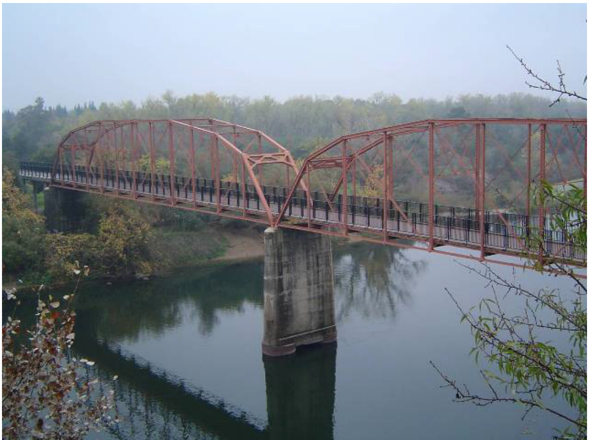
Fair Oaks Bridge
